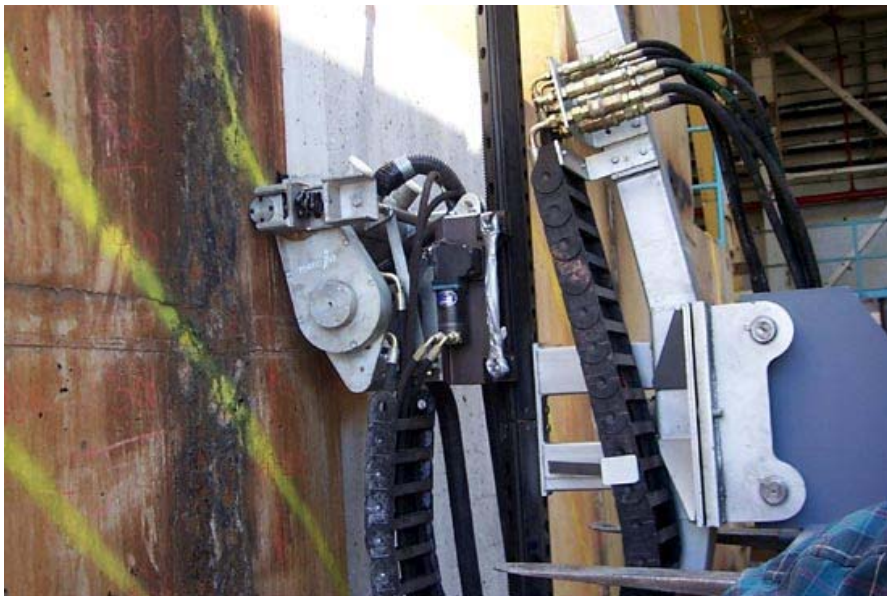
Fig. 1. Concrete shaver decontaminating wall surface.
